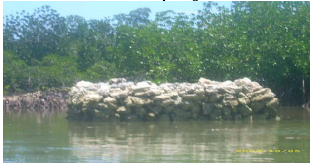
Figure 5.1: A Faurara in its early stages of construction
