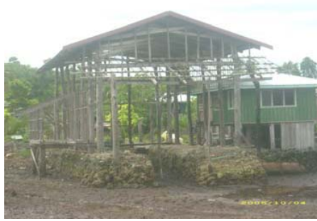
Figure 5.23: A new boat building shed
